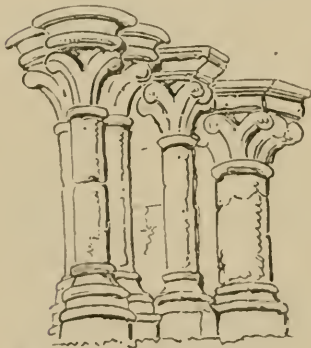
Fig. 58.—Columns at St. Bavon.
